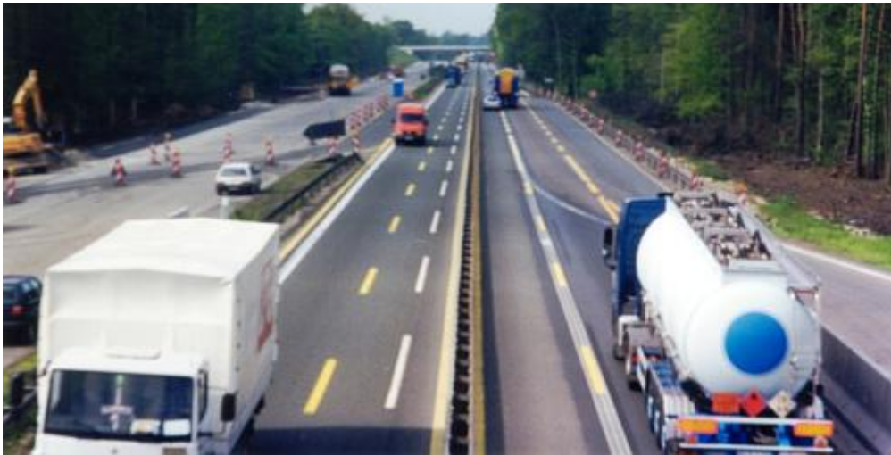
Autobahn construction area. Note the yellow road markings, these supersede all regular markings in work zones.
